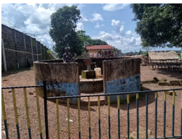
A borehole at the Mafanta CC
