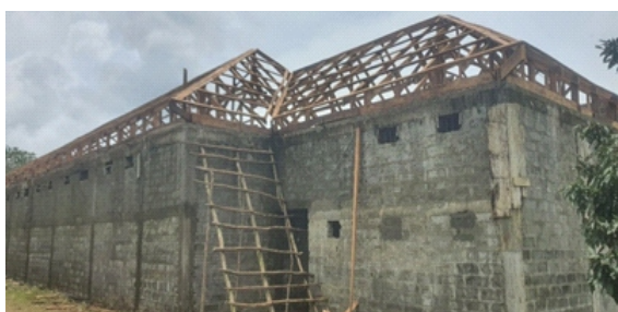
Ongoing construction at the Moyamba CC where male inmates work
